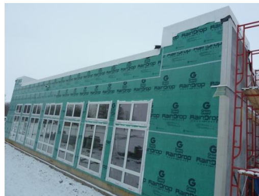
Fig. 2: South wall, March 2011
